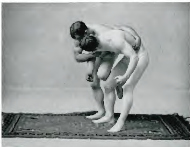
POSITION 43. DRAG HOLD SECURED.
