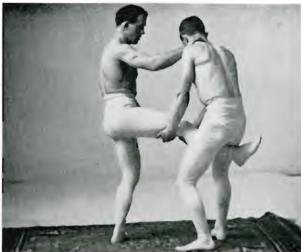
POSITION 55. FIRST GUARD AGAINST THE LEG LIFT.
