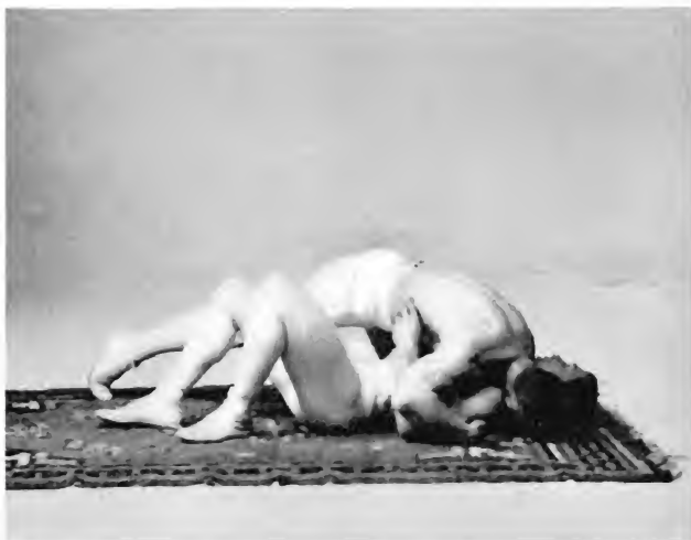
POSITION 150. FALL FROM THE FACE HOLD.
